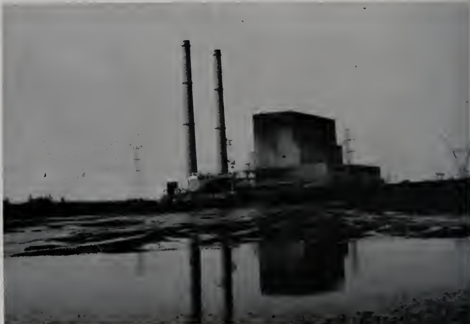
The slag pond adjacent to the Kincaid Generating Station, where waterfowl congregate in the fall.
