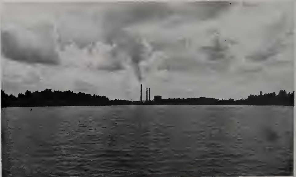
Lake Sangchris and Kincaid Generating Station in 1979, after the construction of a new stack.
