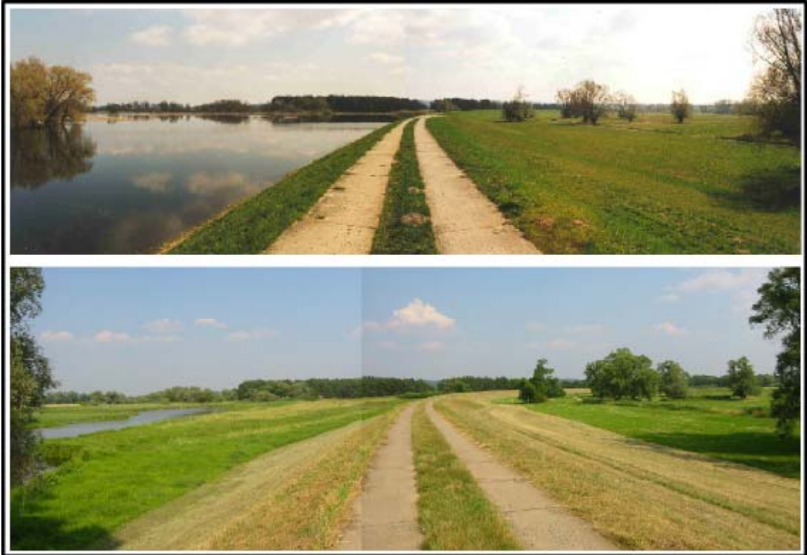
Fig. 3: Management of the flooding regime. “Wet polder” (left) and “dry polder” (right) separated by a dyke. The picture at the top was taken in March, the one at the bottom in July. (Photos: H. Lüssow, J. Rothenbücher)
